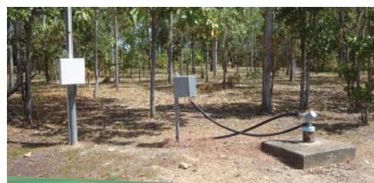
Typical groundwater bore in Howard East area.
